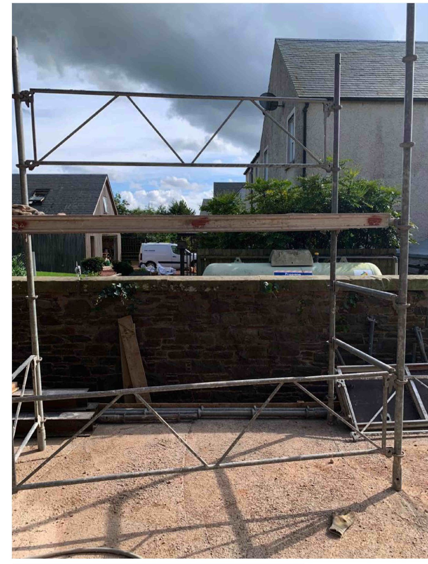
View over boundary wall. Note obstructions - existing gas tank, trees and fencing screen.
